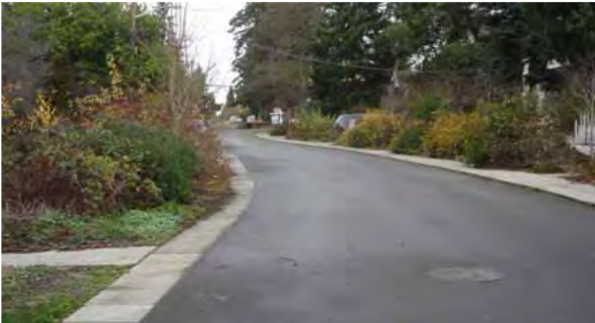
Narrowed travel lane; zero-rise curb; rain garden.
