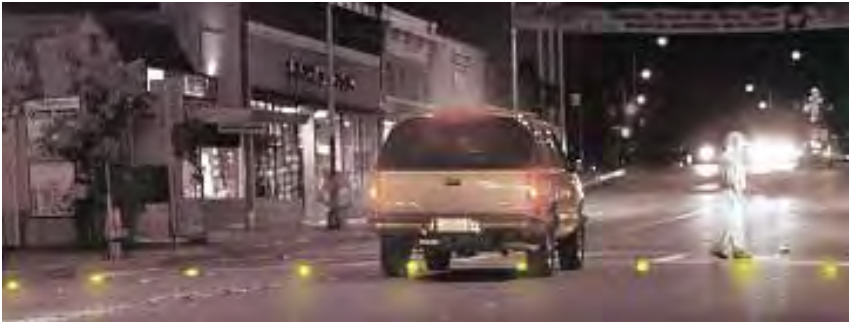
In-pavement lighting is a controversial technology in some communities
