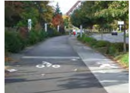
Alert bar warning cyclists of congestion ahead combined with separation of bikes/peds
