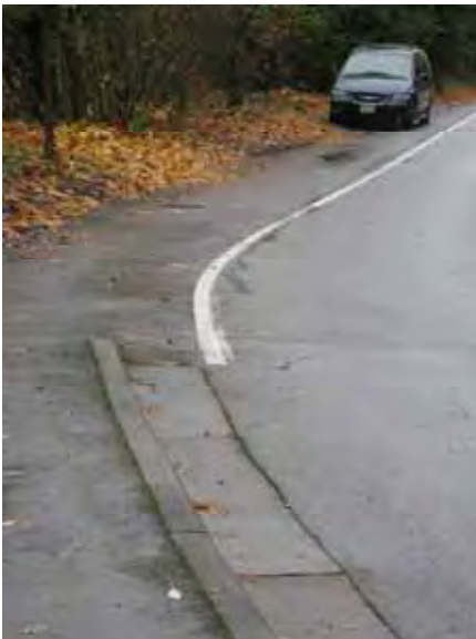
North Mercer Way transitioning between paved shoulder and shared use path
