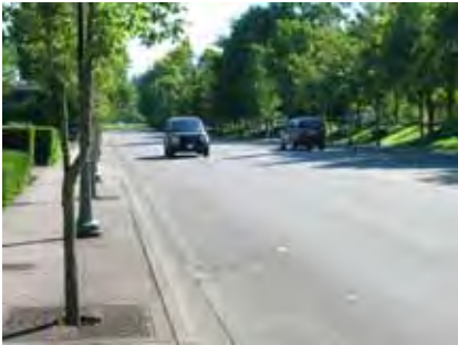
Bike Lane and Sidewalk
