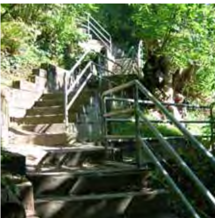
Fleury stairs provide multiple connections, and opportunity for views and seating.
